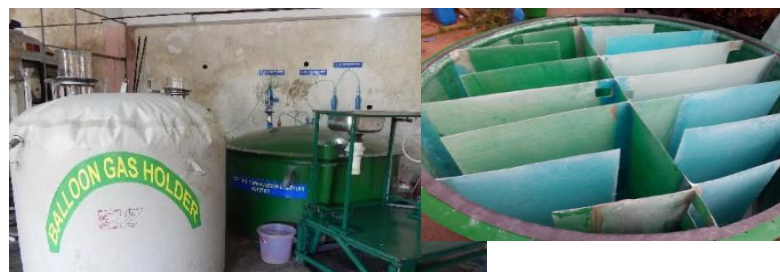
Rumen model biogas plant
